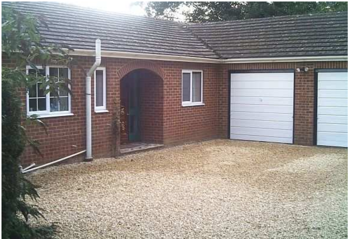
The driveway, garage and front-door to Merry Meeting
